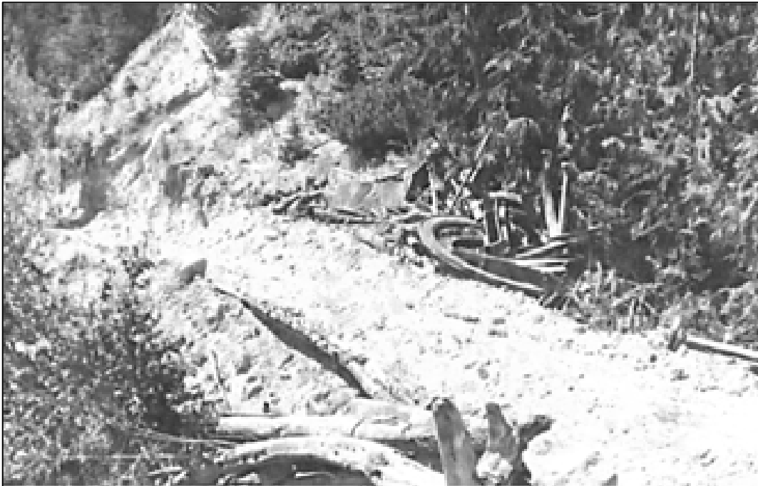
Figure 3.30. Ore Concentrator Parts beside Remains of the Storbo-Glacier Basin Road. (Photograph taken in 1952 by Douglas Evans. In NARA Archives L3023 Files Box 50 Folder 60)
