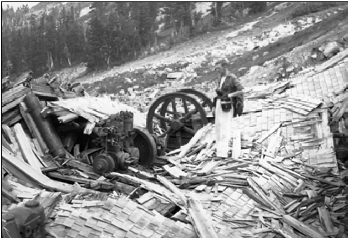
Figure 5.10. P.T. Storbo's Son, Albert, Surveys Reven Mine Remains in 1956. (Courtesy Arthur L. Storbo)
