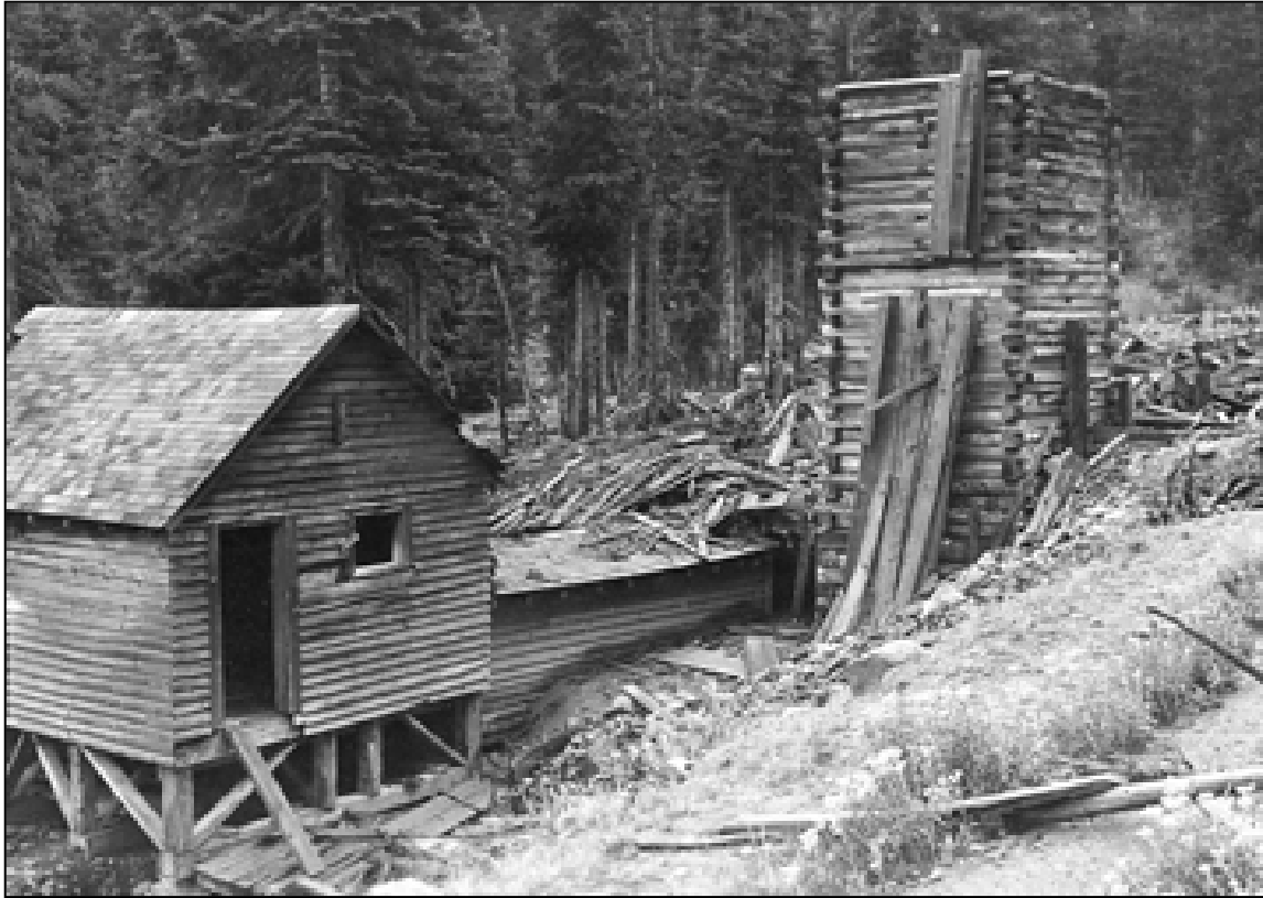
Figure 4.11. Glacier Basin Generator and Saw Mill ca. 1951.
